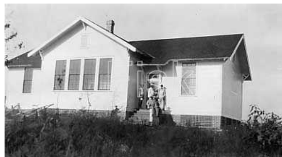
Arcola School, Hale County, Alabama, built 1923-24
